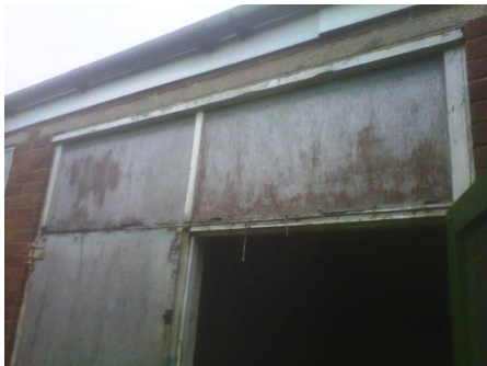
Dilapidated framing and dislodged fascia.
